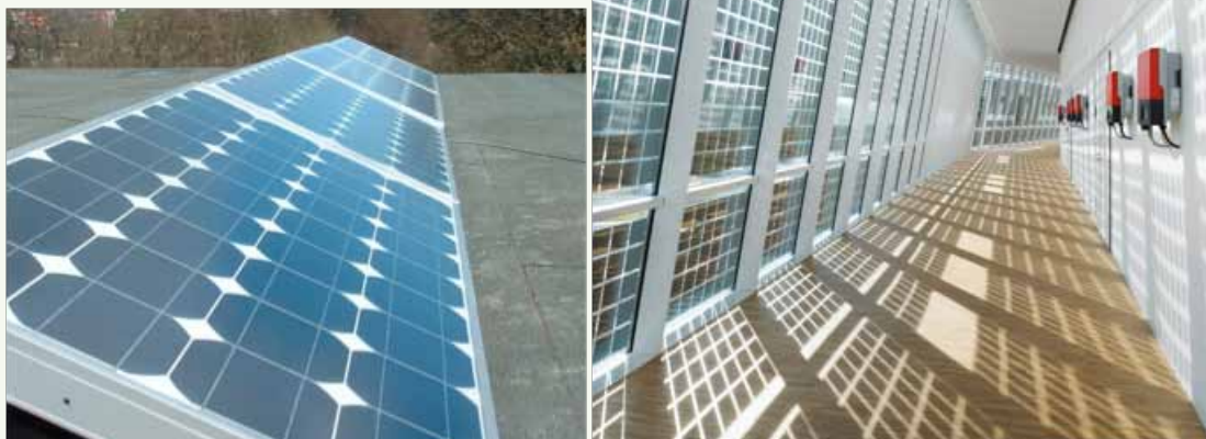
Figure 35: BAPV (Left) and BIPV (Right) Systems
