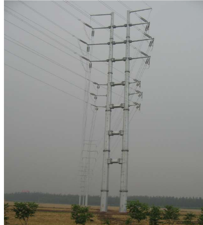
(B) MONOPOLE WITH MULTI CKT & MULTI VOLTAGE
