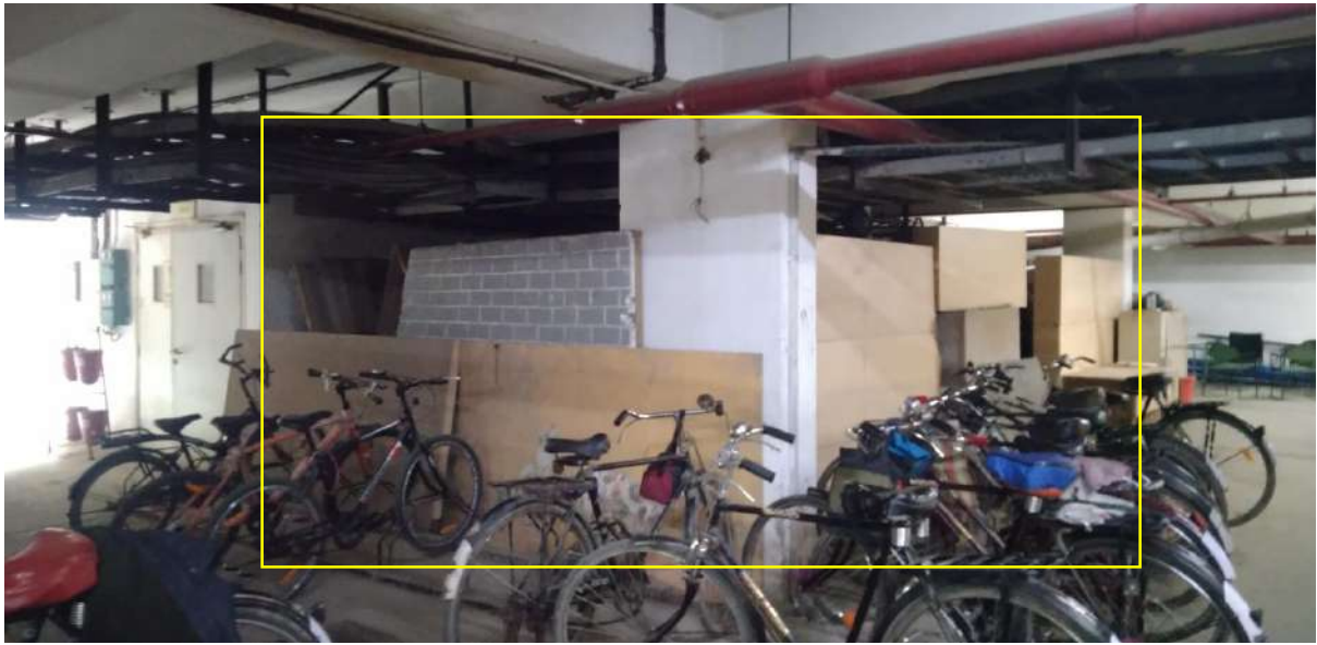
View of space for BESS installation, cable trays, debris present
