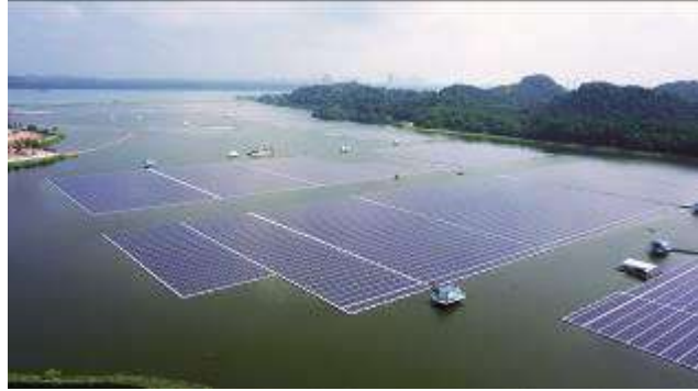
Photo 1a: Aerial View of the Sembcorp Tengeh Floating Solar Farm
